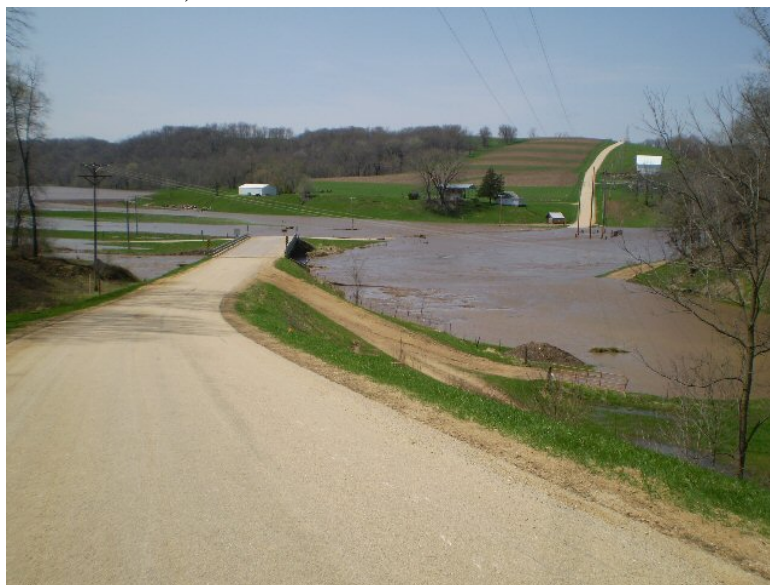
Figure 2: Camel Ridge Road Overtopping, Waterloo Township - April 25, 2008 Flood (Reference 12)
